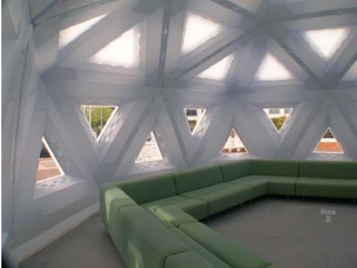
DecaPod interior with translucent windows above and Plexiglas windows below
