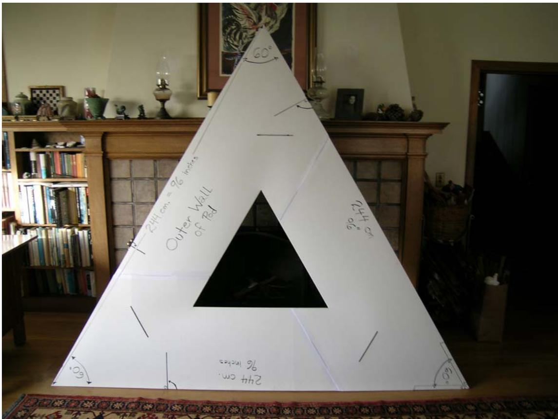
All of the DecaPod wall triangles are equilateral. The outside edges of the triangle
