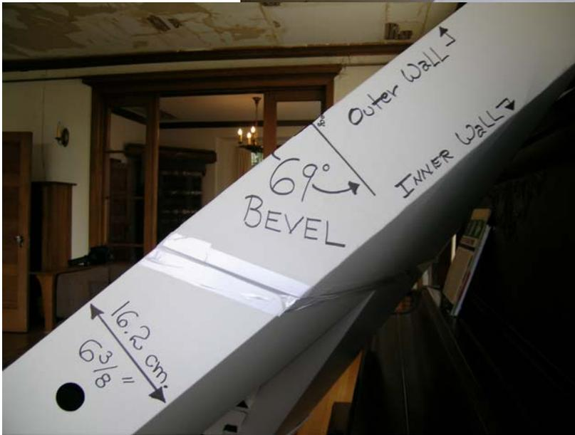
outside wall. Thus the edges that create the 6" (15.24 cm) thickness of each of these triangular "doughnuts" are not perpendicular to the inside and outside edges, but actually bevel
