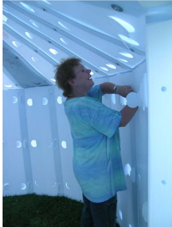
Circular access holes in the Yurt wall and roof components make it easy to bolt the components together and later pack them with straw or other insulating material.
